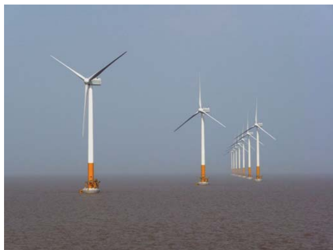
Sinovel's 3 MW Wind Turbines in Shanghai Harbor
